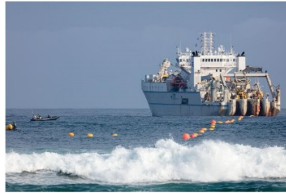
Picture 2: Submarine cable laying in progress
